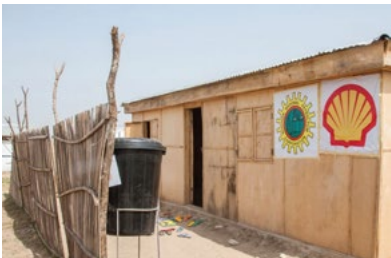
↓ Newly constructed safe-place
